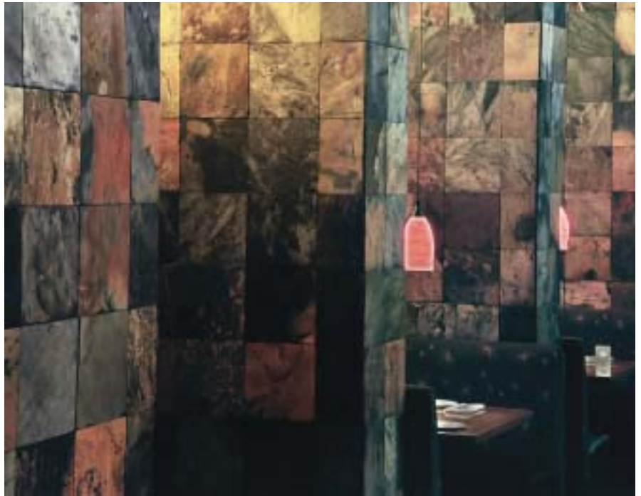
While builders might find a place for slate as a flooring accent near a doorway or on an outside patio, architects find the variation in the stone's look can make for an interesting wall cladding.
