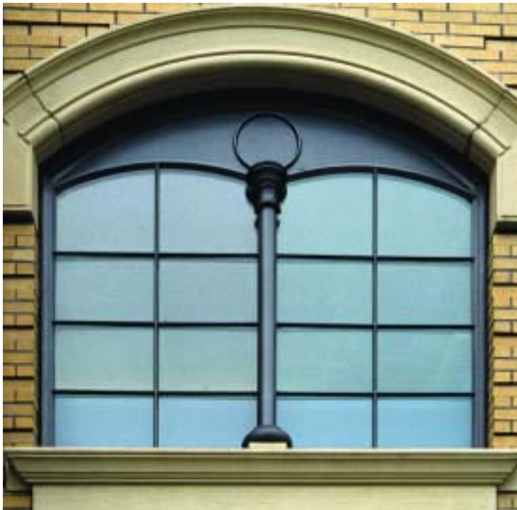
For architects, it's not always an either/or situation. At the San Francisco Wax Museum, natural stone with window fittings and copings worked well with standard brick-type masonry
